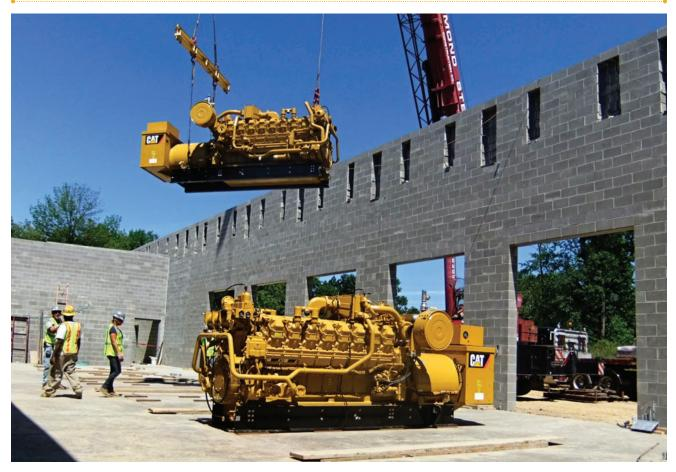
These enormous CAT engines will utilize landfill gas to create electricity at a new Landfill Gas to Electric plant.
