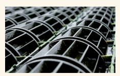
Algaewheels grow algae in a controlled environment. In turn, algae produce oxygen, which bacteria in the system use to convert wastewater organics into carbon dioxide.
