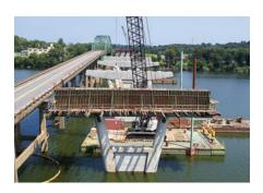
The new bridge is a composite deck slab bridge with precast, prestressed 72" bulb-tee beams and welded steel girders. It will have four lanes, eight piers, and be 1,616 feet long.
