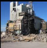
RIGHT: Environmental investigation, mitigation, and demolition activities for numerous multi-unit boiler houses, ancillary structures, and equipment at six retired generation stations in Ohio.
