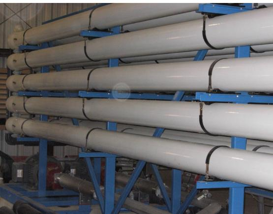
The AWTP is a new wastewater recycling process that utilizes a combination of reverse osmosis, microfiltration, and a fully automated proprietary process to recycle more usable water and generate less reject water than standard reverse osmosis or multi-stage reverse osmosis with chemical treatment.
