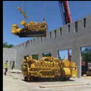
TOP: On-site 100,000-gallon-per-day leachate pretreatment facility in Murfreesboro, Tennessee.
